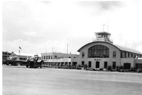
1928 Miami International Airport
