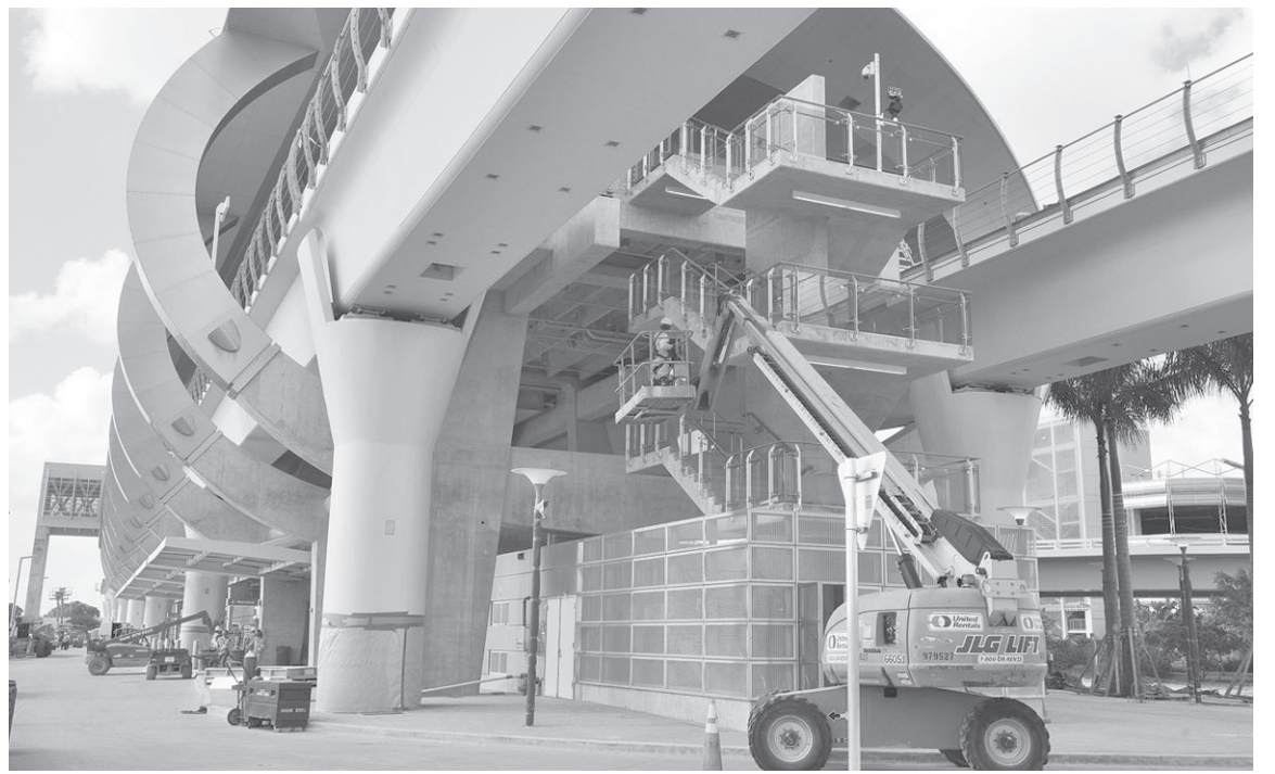
Work continues at the Metrorail and Metrobus station component of now-rising Miami Central Station.
