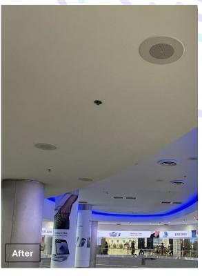
• Repair of the tear drop ceiling areas caused by roof leaks on the second floor of MIA's North Terminal by Door No. 8.
