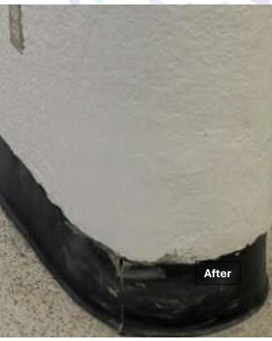
Repair of damaged column due to smart-carts, golf carts and other luggage on the second floor of MIA's Central Terminal by Door No. 17.
